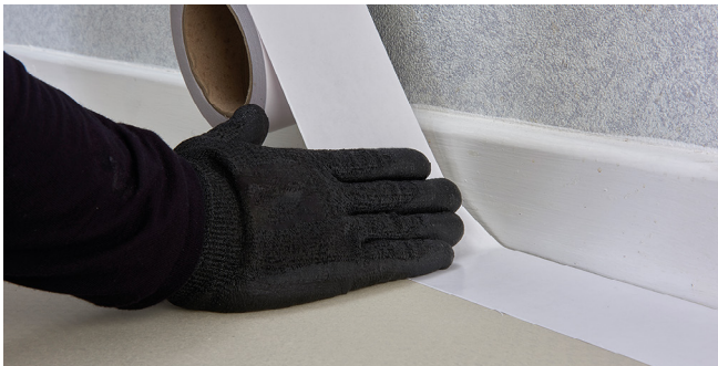
Figure 12 Use double sided Polyflor recommended tape
