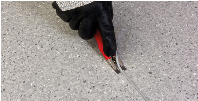
Figure 4b Trimming off the weld top layer (Mozart Trimming Tool)
