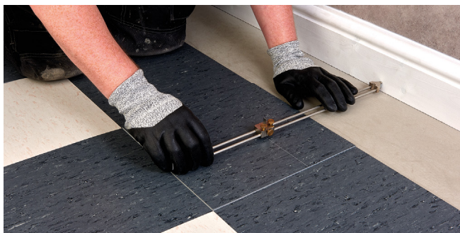
Figure 6 Measuring a tile using a scriber
