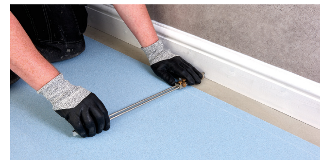
Figure 2 Scribing the wall profile
