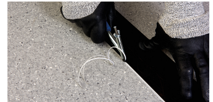
Figure 1 Grooving the seam
