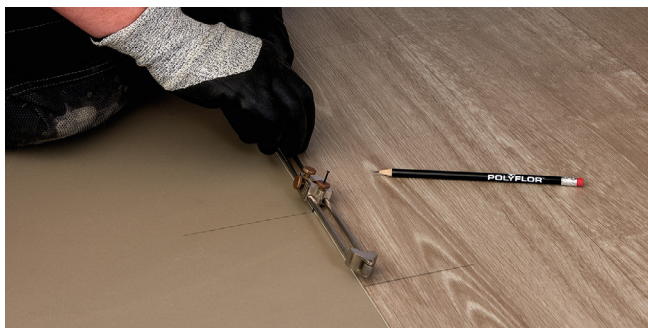
Figure 4 Scribing the wall profile
