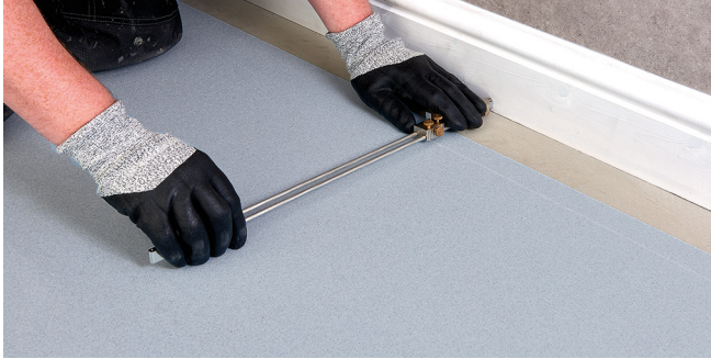
Figure 11 Scribing the wall profile
