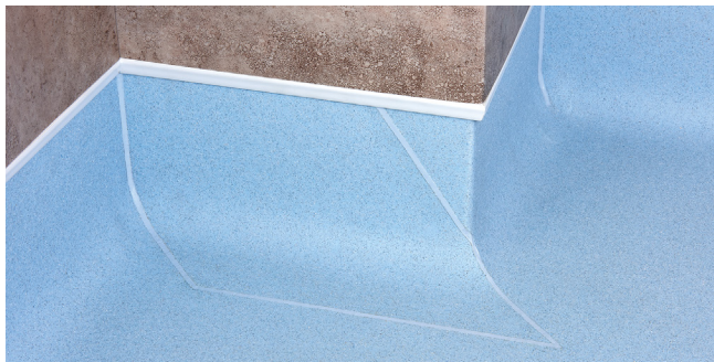
Figure 11 External corners 'wrap around method'
