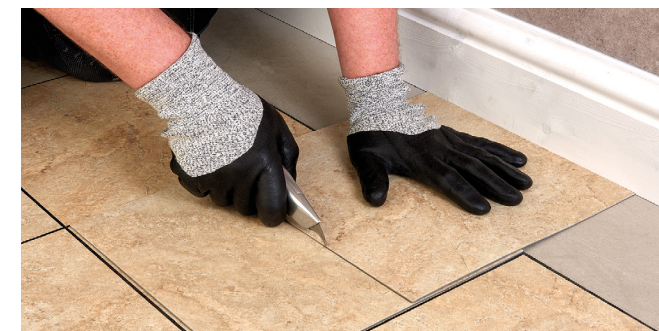
Figure 6 Measuring using an overlapping tile
