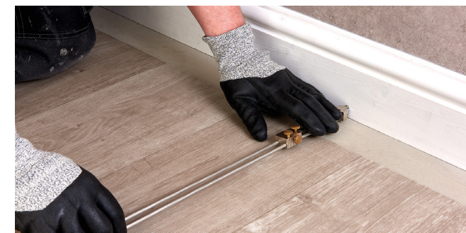
Figure 2 Scribing the wall profile
