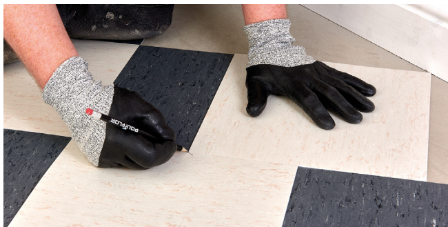
Figure 7 Marking the perimeter tiles (diagonal cut)
