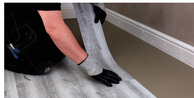
Figure 1 Setting planks out
