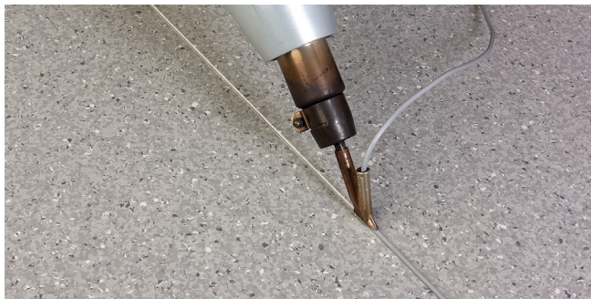
Figure 2 Applying the weld
