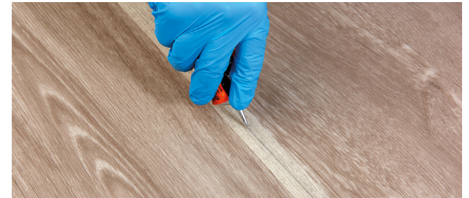
Figure 7 Cold welding
