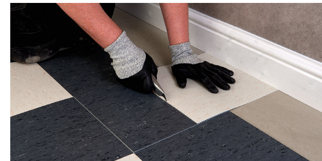
Figure 5 Measuring using an overlapping tile
