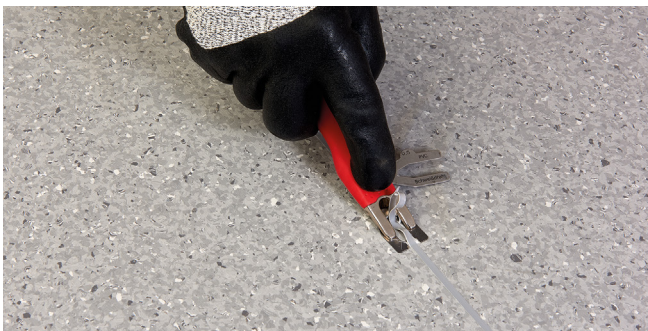
Figure 5b Final trim after the weld has cooled (Mozart Trimming Tool)
