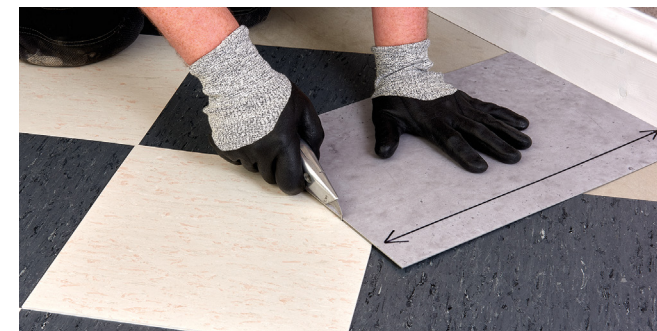
Figure 8 Cutting the perimeter tiles (diagonal cut)
