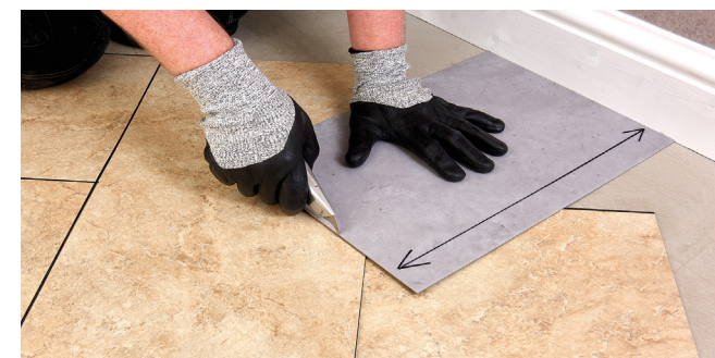
Figure 9 Cutting the perimeter tiles (diagonal cut)
