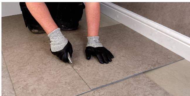
Figure 8 Measuring using an overlapping tile
