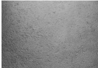
Basalt stone structure
